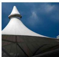
The structures are all prefabricated to engineered drawings and calculations, with some membranes being as large as 1000 sq.m before reaching site. The size of the overall structure can be relatively unlimited when employing site joints. Applications include: entrances, walkways, features, sports stadia, atria, retail, exhibitions, and landmarks.
