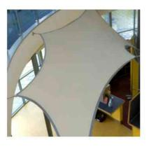
The membrane is an extra strong, aerated textile that is corrosion-proof and easy to maintain. It offers the possibility of playing with light, materials and shapes, giving volume and colour to the ceiling. Installation is made easy using our modular ceiling panel system, by combining extrusion jointing and then tensioning using calibrated stainless steel traction springs on the outside fabric boundaries
